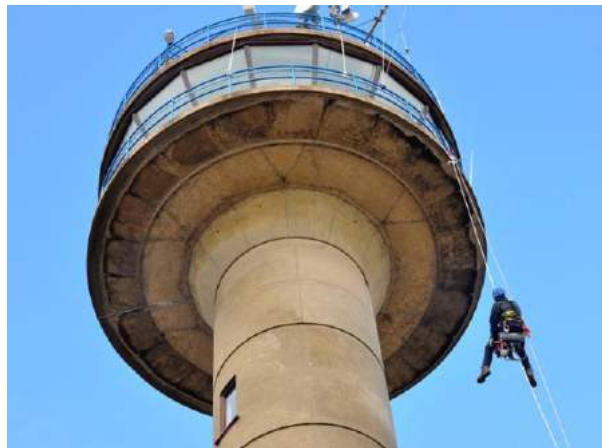
Alternative ways to access the Calshot Tower operations room: (left) Hampshire Fire and Rescue high rise platform; (right) A motorised bosun's chair.
