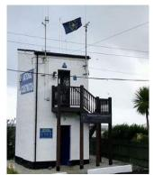
A few years later, an external staircase was added to the tower to improve the safety of the watchkeepers when accessing the lookout on the top floor. This staircase also has observation platforms so visitors can observe the whole of Mounts Bay.
