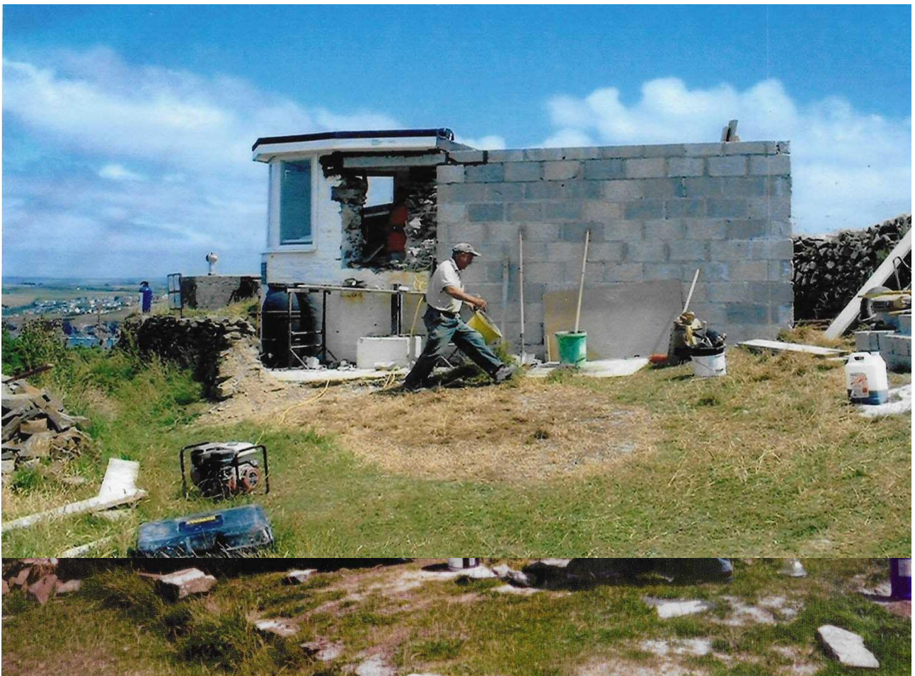
Initial restoration of the lookout
