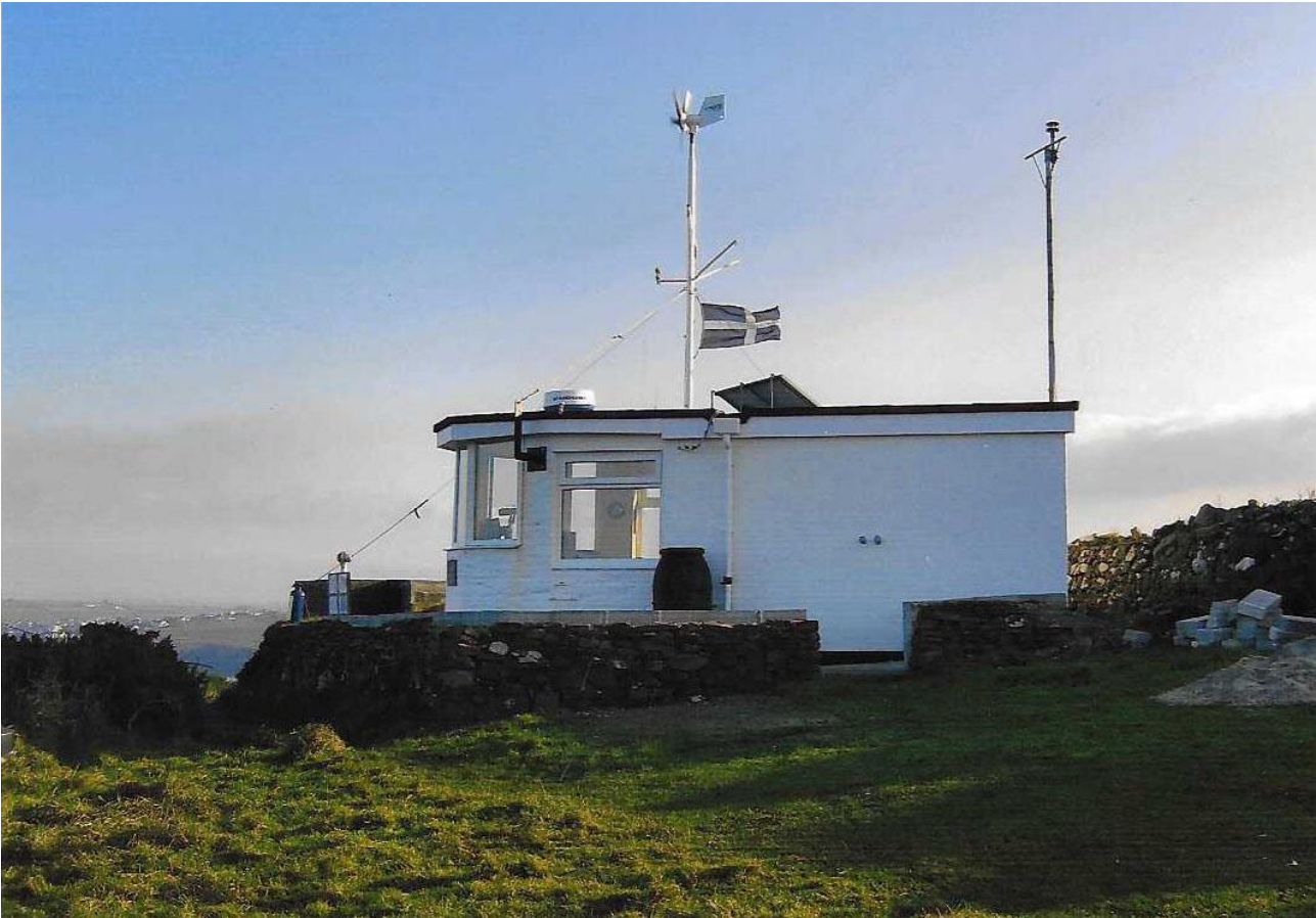
Completion of second restoration
