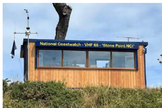
The new NCI Stone Point station arrives, is fitted out, and brought into use
